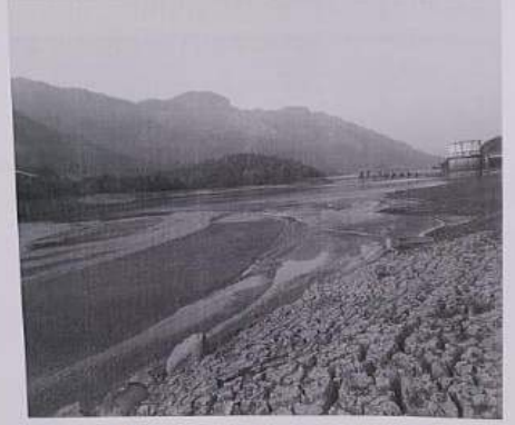
OF PILLUR DAM.
